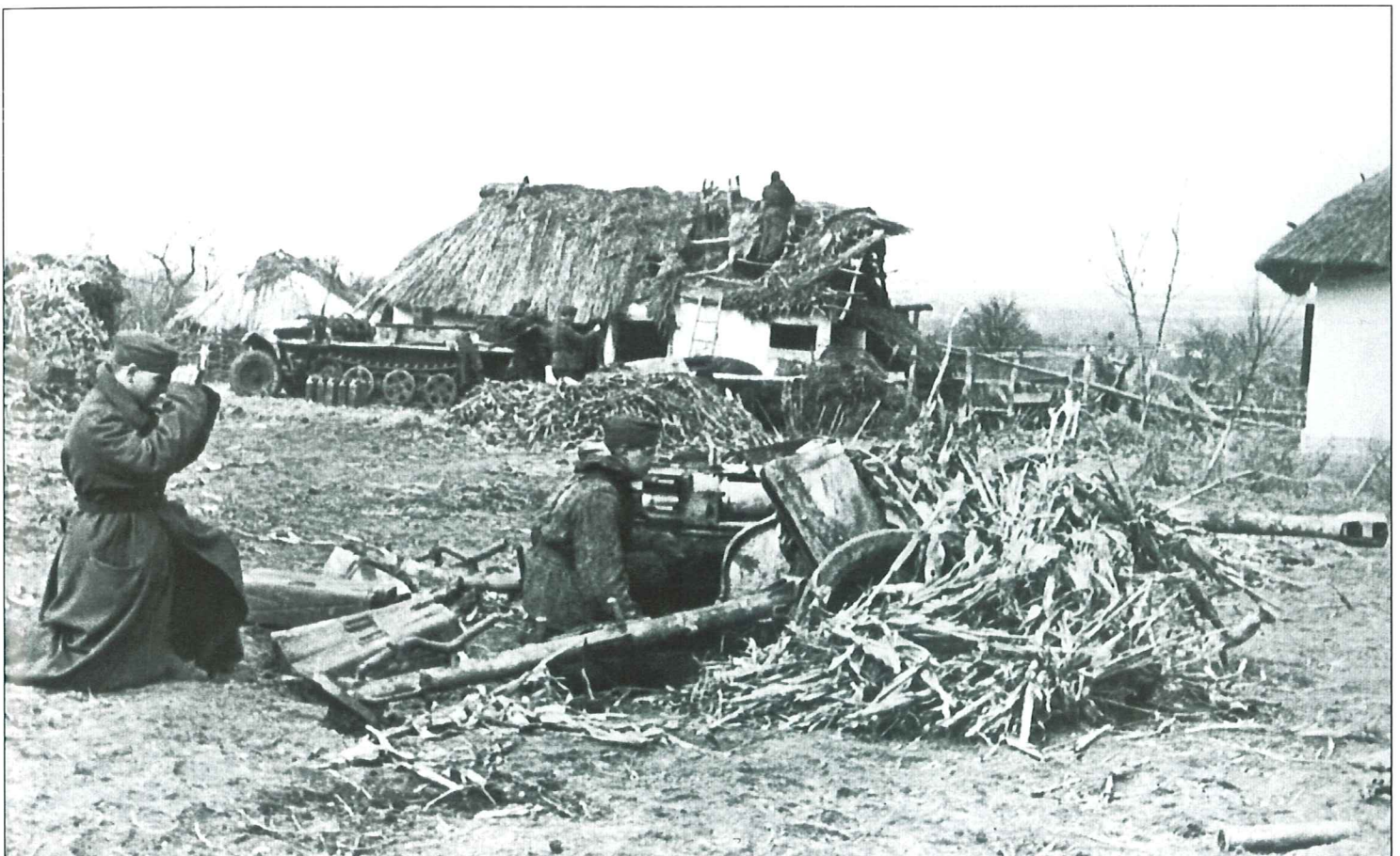
A 5cm PaK 38 anti-tank gun manned by SS troops waiting in a camouflaged position on the southern sector of the Eastern Front, somewhere in the Ukraine. In the background is an Sd.Kfz.10 with another Pak 38 behind it. The photo was taken in the late spring of 1944, however, the half-track and guns still show signs of their white winter camouflage paint. Note the observer on the roof of the farmhouse beside the Demag.
