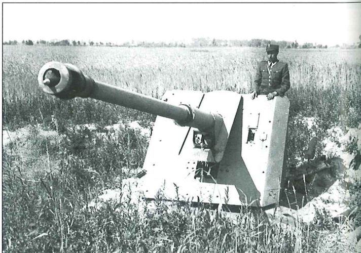
As carefully dug in as it is, this 8.8cm PaK 43.L/71 would be nearly impossible to detect from a distance. The PaK 43 was the finest anti-tank gun produced during WWII and was issued to frontline troops in time to deal with the new Soviet JS-2 tanks appearing on the Eastern Front in late 1943. It was transported on a cruciform carriage developed from the 8.8cm anti-aircraft guns and ran on four wheels. Air raids on the factories resulted in a lack of carriages and a slightly different version of the gun was mounted on the carriage of the 10.5cm leFH 18 with the wheels from the 15cm sFH 18 resulting in the towed version of the gun, the 8.8cm PaK 43/41.L/71.
