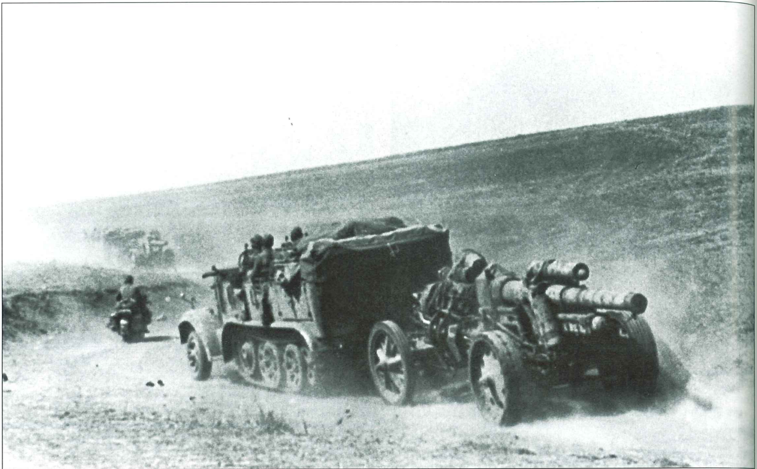
An Sd.Kfz.7 towing a 15cm sFH 18 howitzer across the steppes in the Stalingrad area, September 1942. In the background, another similar artillery team can be seen. Note the sand colored camouflage pattern on the gun barrel applied over the dark gray background.
