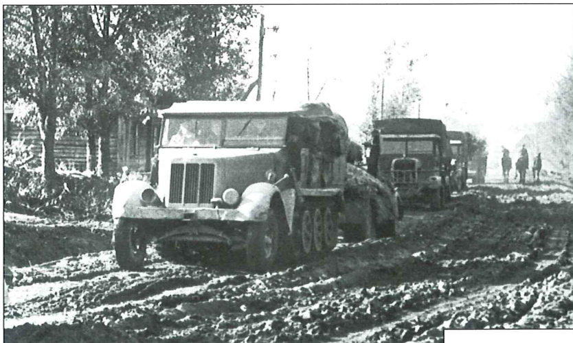
An Sd.Kfz.7 towing a 15cm sFH 18 howitzer across the steppes in the Stalingrad area, September 1942. In the background, another similar artillery team can be seen. Note the sand colored camouflage pattern on the gun barrel applied over the dark gray background.
