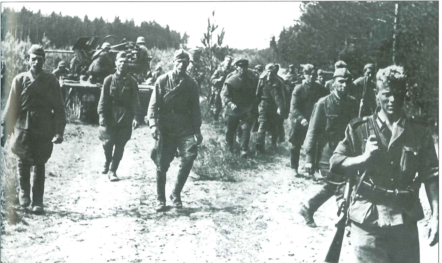
During an early period of the war in the Soviet Union in 1941, a group of Soviet POWs are being marched into captivity, passing near an Sd.Kfz.10/4 with its 2cm FlaK 38 fully depressed to engage ground targets. The FlaK 38 was very useful against light armored targets because the armor piercing Pz.Gr.40 could penetrate 20mm plates at a range of 500 meters.
