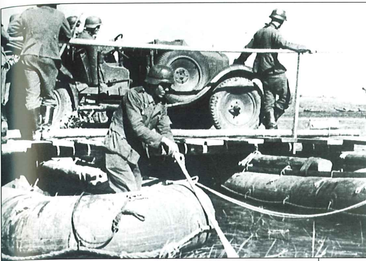
A pontoon ferry crossing a river in Russia in 1941 with a Mercedes-Benz Stuttgart Kfz.11 or Kfz.12 on board. The first mass produced cross-country car of its type produced for the Wehrmacht, it was old and obsolete when WWII began. Vehicles of this type, about nine models, were too big and did not have the good cross-country capabilities of their successor, the Kübelwagen, or their United States counterparts, the Willys Jeep.
