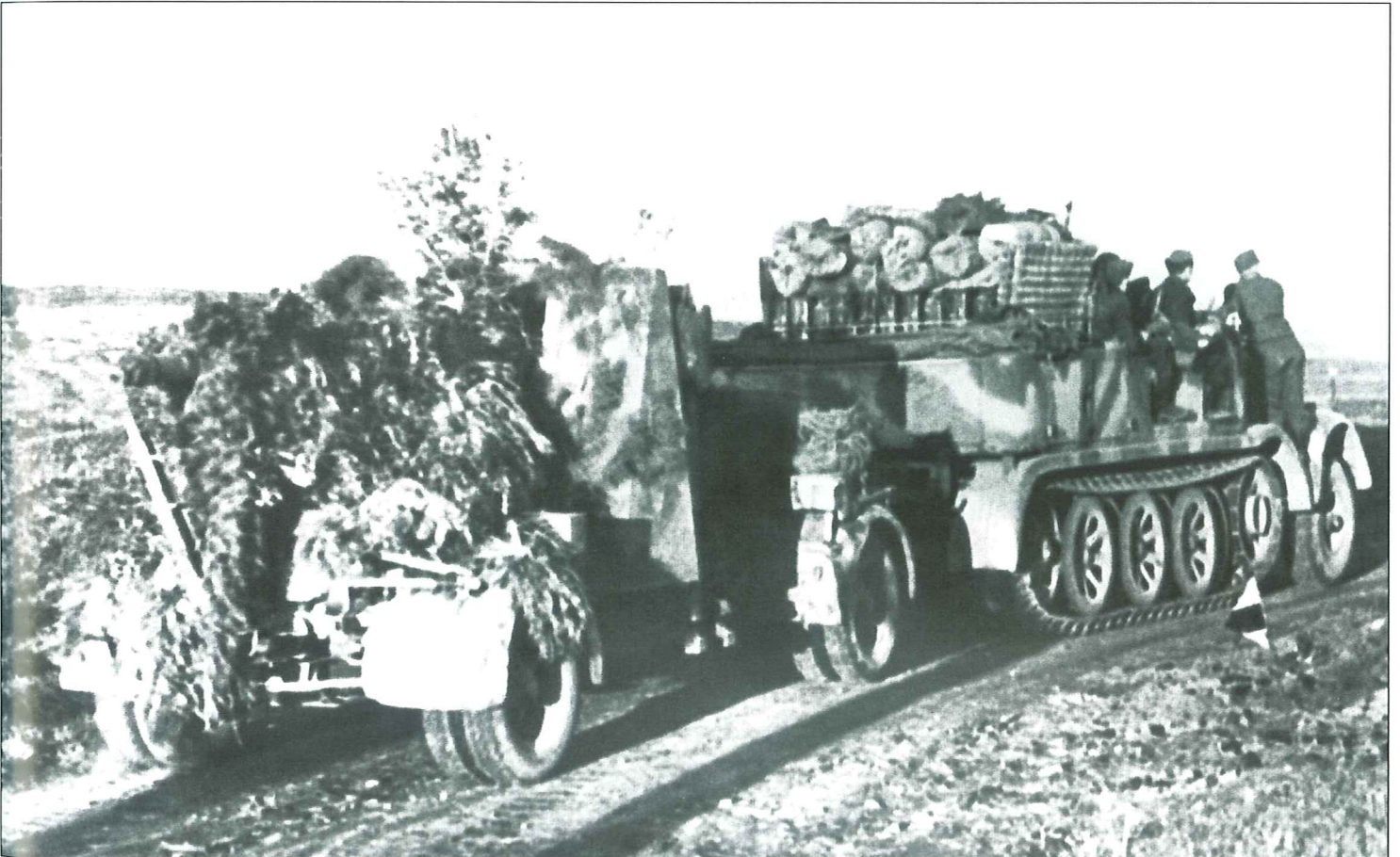
A Sd.Kfz.8 loaded with the personal gear of the crew and 10 additional jerry cans, towing a heavily camouflaged 8.8cm FlaK 36/37 anti-aircraft gun across the expanses of the southern Soviet Union in the late summer or early autumn of 1942. The half-track is painted with a camouflage pattern that was standard for Wehrmacht vehicles at the time. It is composed of an irregular sand color applied on the sides and top of the vehicle. Introduced in the early summer of 1942, it was intended to break up the very dark, solid gray shape of the vehicle. Note the divisional HQ command pennant stuck in the ground beside the road.
