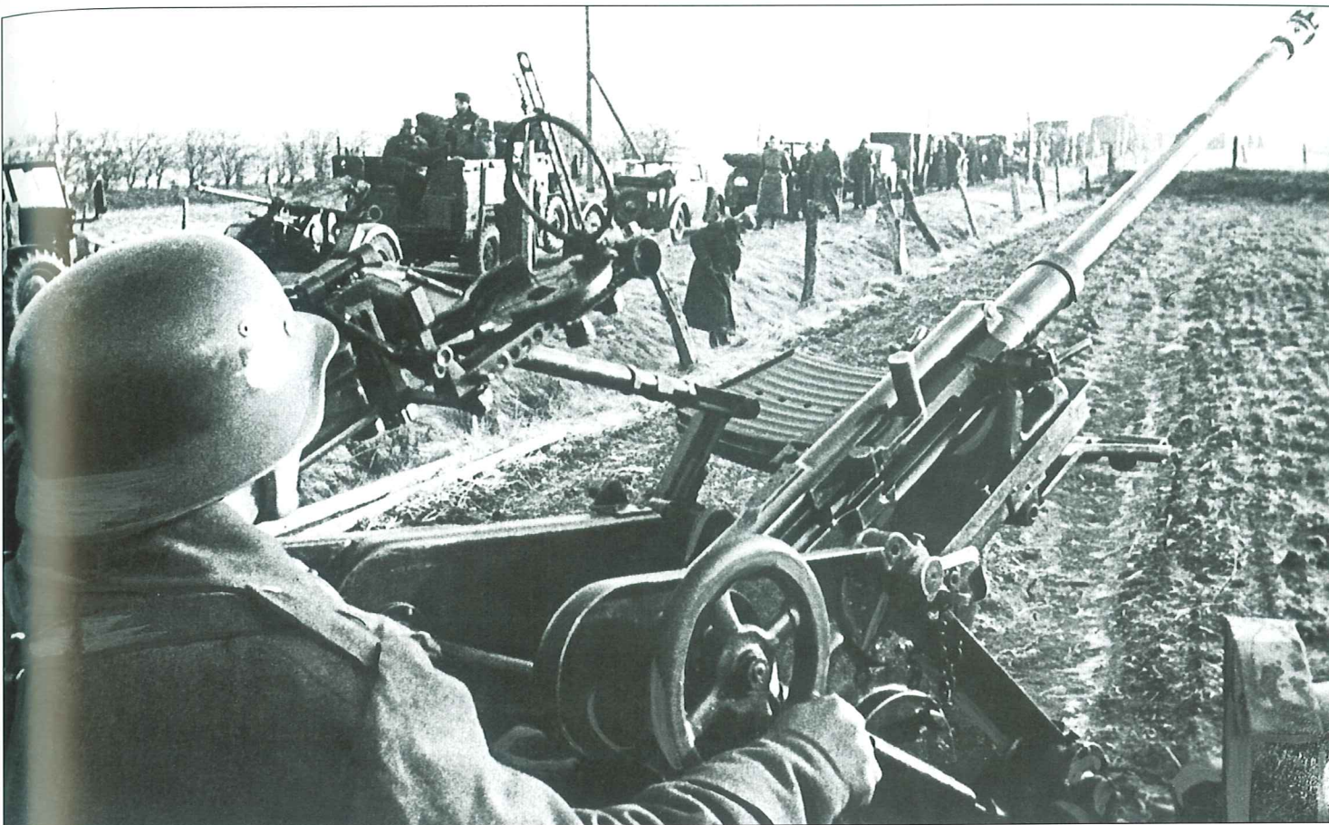
A column of cars and trucks during a march break, probably somewhere in Western Germany during the early stages of the war. The column is guarded by a 2cm FlaK 30 light anti-aircraft gun while other similar weapons are being towed by the Krupp Protz Kfz.69 in the background. This was the most common type of towing vehicle during this period and was replaced by the heavier Horch 1a later on. Note the details of the 2cm gun and sight in the foreground.
